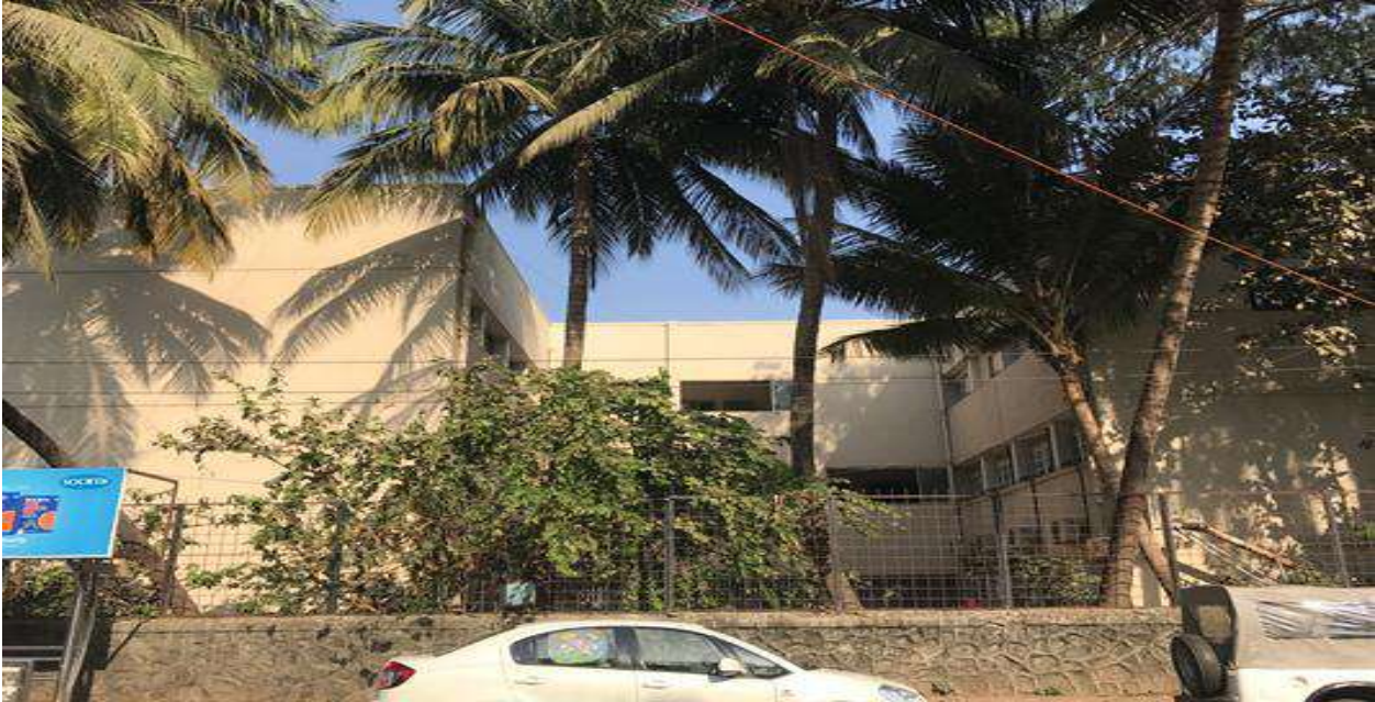
PH NO-06:-Photograph showing the existing view of structure.
