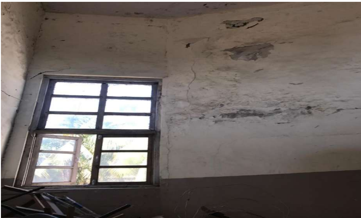
PH NO-50:-Photograph showing structural crack on column at second floor staircase area.
