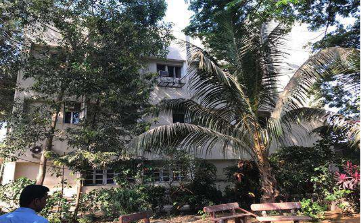
PH NO-09:-Photograph showing the existing view of structure.
