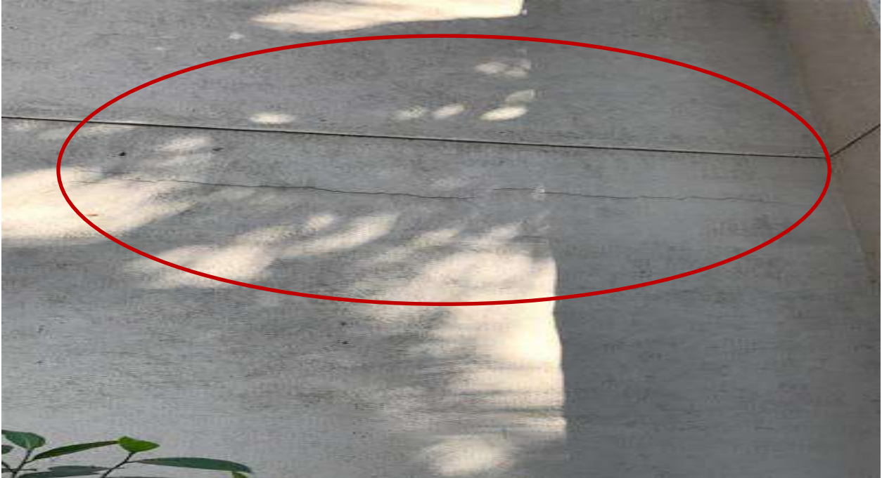
PH NO-04:-Photograph showing separation crack between beam and wall.
