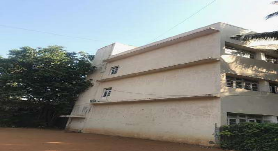
PH NO-18:-Photograph showing the existing view of structure.
