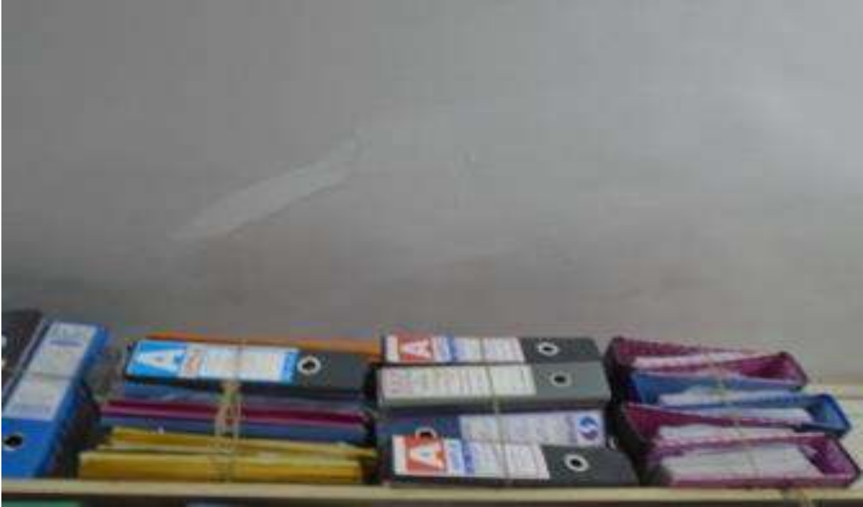
PH NO-17:-Photograph showing bulge concrete cover on slab at office no- 32.
