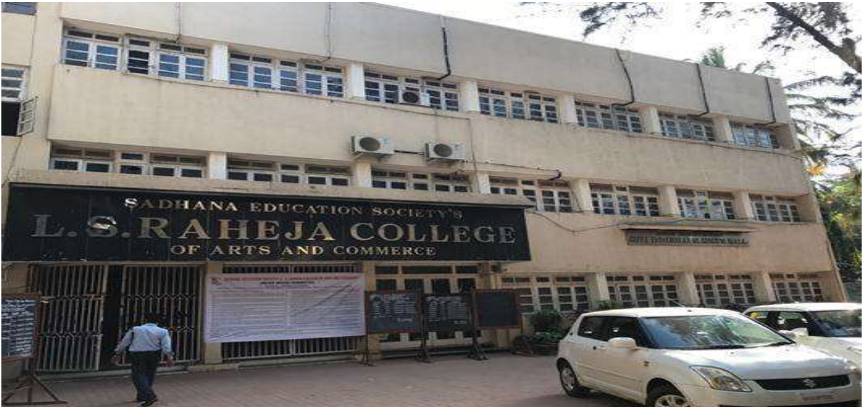
PH NO-01:-Photograph showing the existing view of structure.
