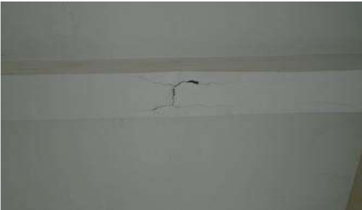
PH NO-24:-Photograph showing bulge concrete cover on beam bottom.
